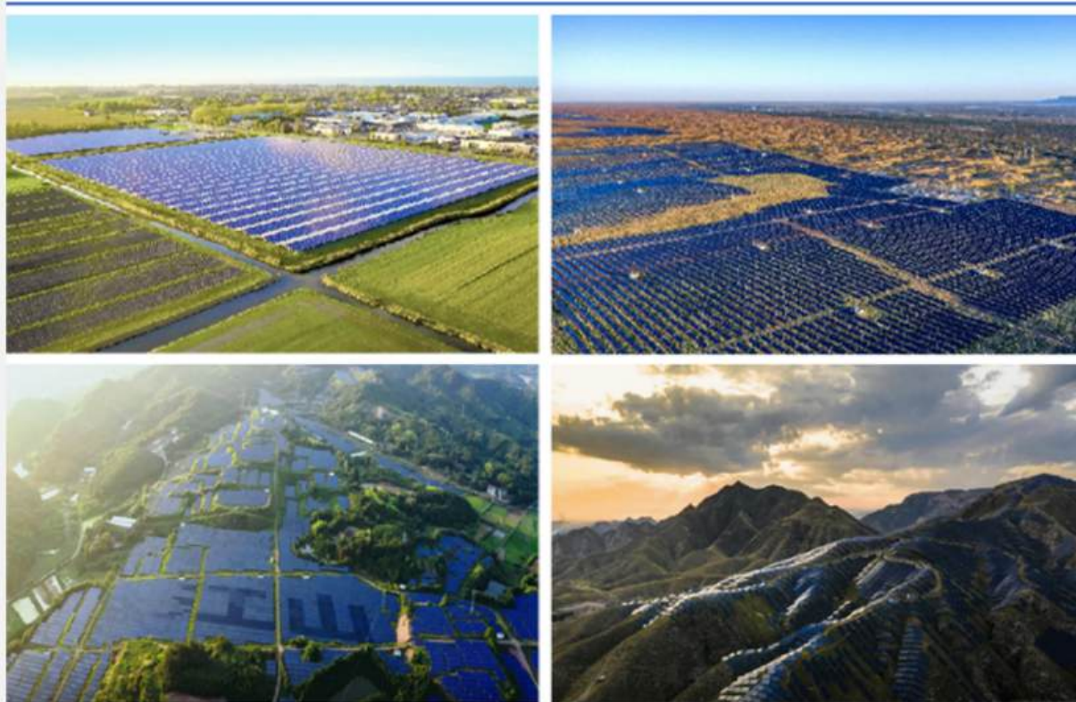
Figure 8: CHINT Global Photovoltaic Power Station Projects
