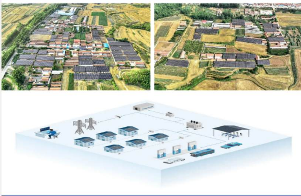
Figure 6: CHINT Aneng Whole Village Development and Smart Microgrid
